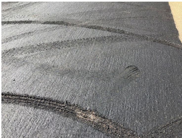
Figure 24: Early traffic damage
