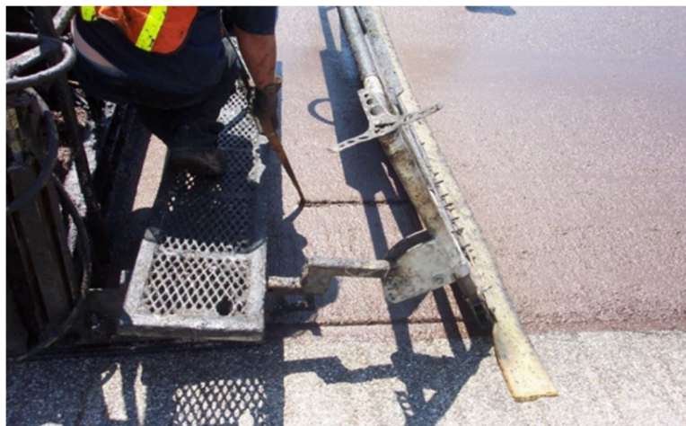
Figure 14: Secondary strike off correcting drag marks
