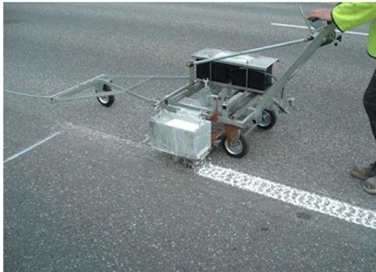
Figure 8: Grinding thermoplastic pavement markings
