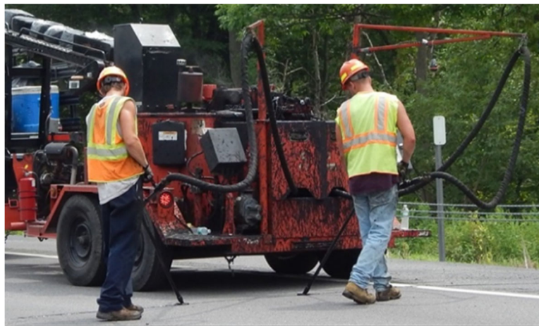
Figure 4: Crack Sealing
