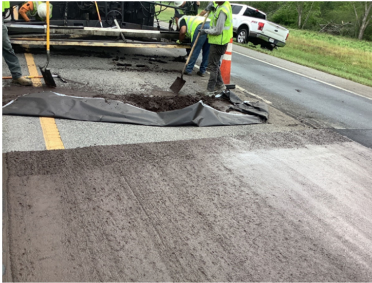
Figure 20: Correct transverse joint
