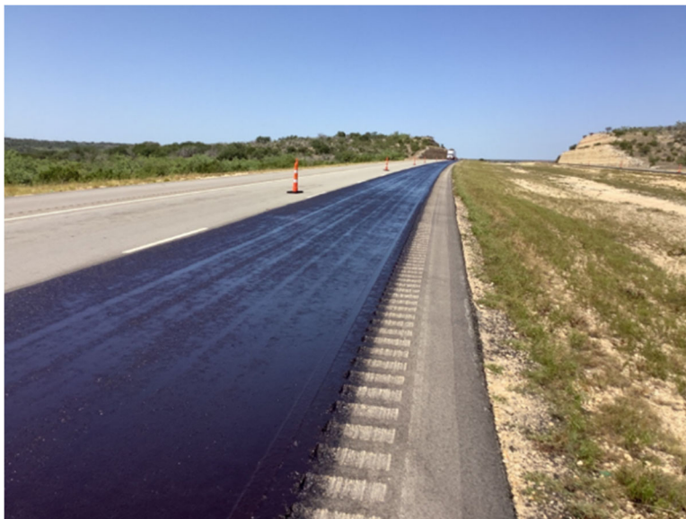
Figure 12: Tack coat before micro surfacing is placed
