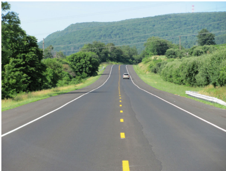
Figure 19: Unacceptable longitudinal joint
