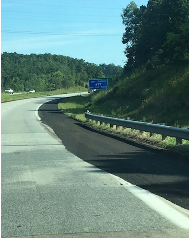
Figure 23: Unacceptable edge line
