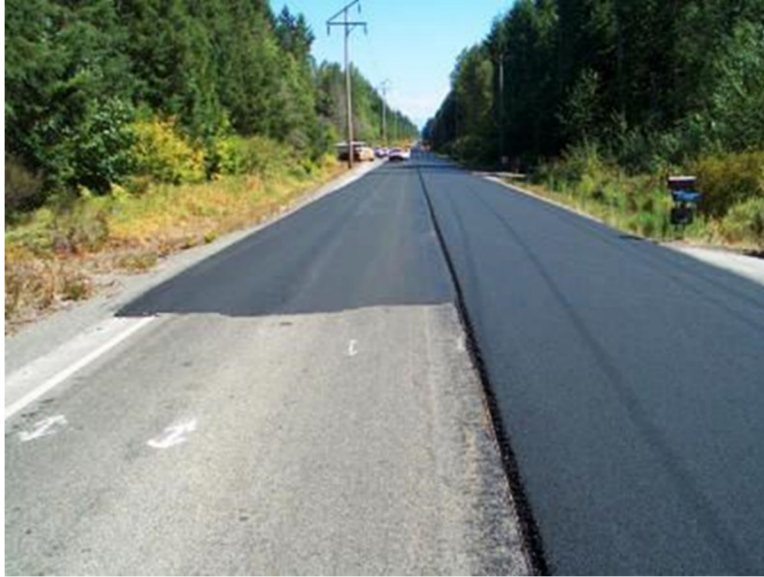
Figure 5: Structural Leveling
