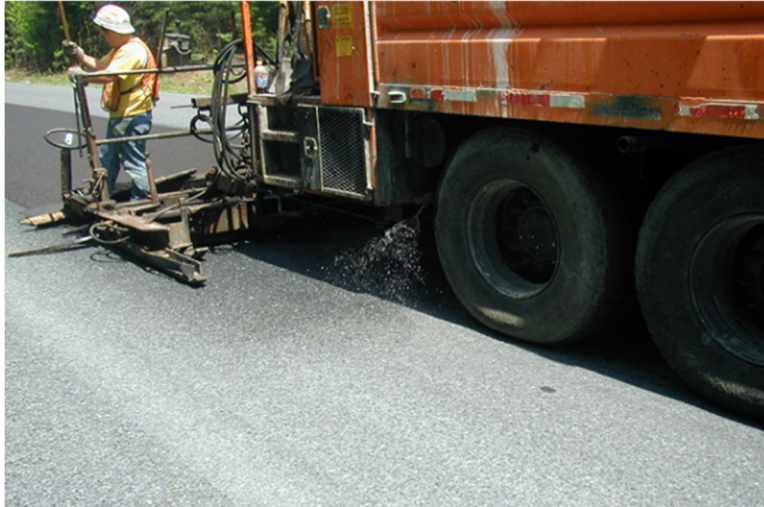
Figure 11: Pre-wetting the pavement prior to placement
