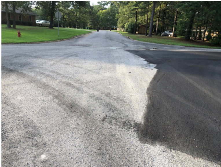
Figure 21: Unacceptable transverse joint
