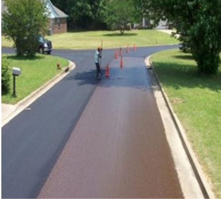
Figure 18: Good longitudinal joint
